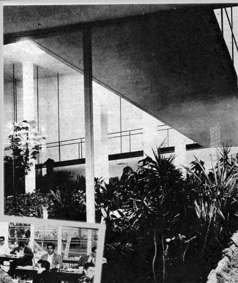
Pride of the Pius XII House of Exercises is the magnificent ramp that facilitates access to the upper floor.
